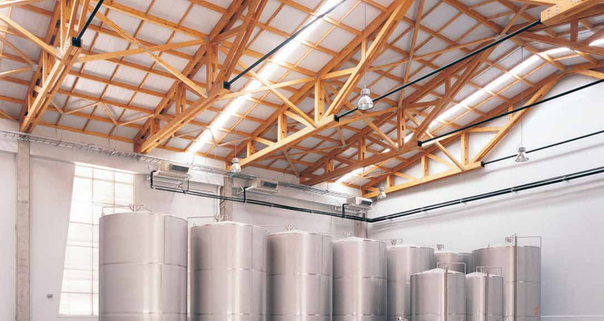
Olisur Olive Oil Factory – Guillermo Hevia – La Estrella, Chile
